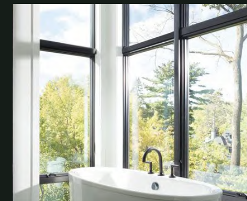
External Doors & Windows Powder Coated UPVC and Glass
